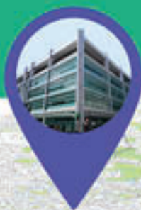
UCLH - FGA building (Maternity Ward)
