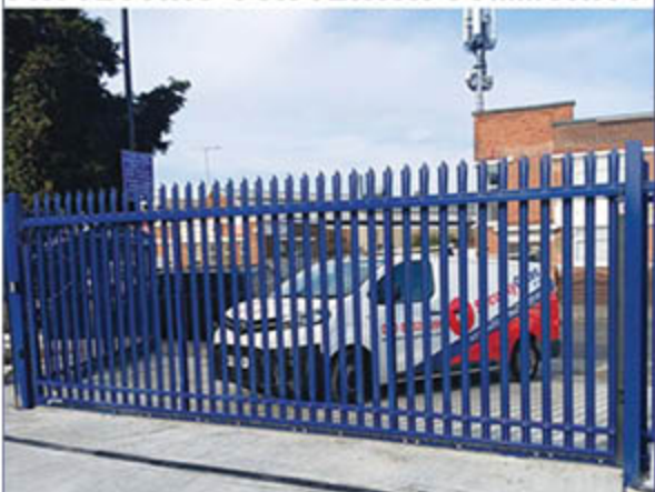
Commerical Automated Palisade Sliding Gate
