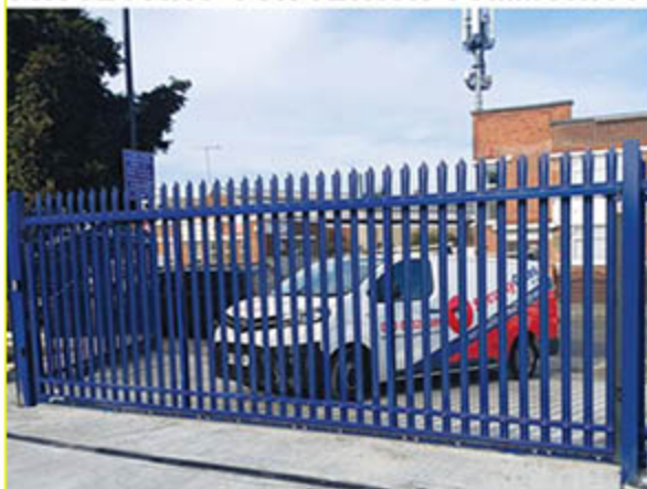
Commerical Automated Palisade Sliding Gate
