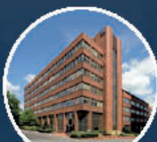
75,000 ft² Office Building Basingstoke
